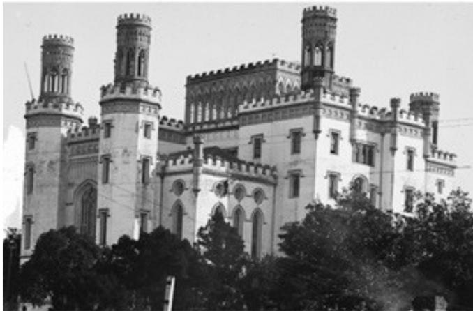
Chicago City Hall and County Building, built 1885. It suffered from structural defects with its foundation that caused the building to sink, and was later replaced with the current City Hall in 1931.
